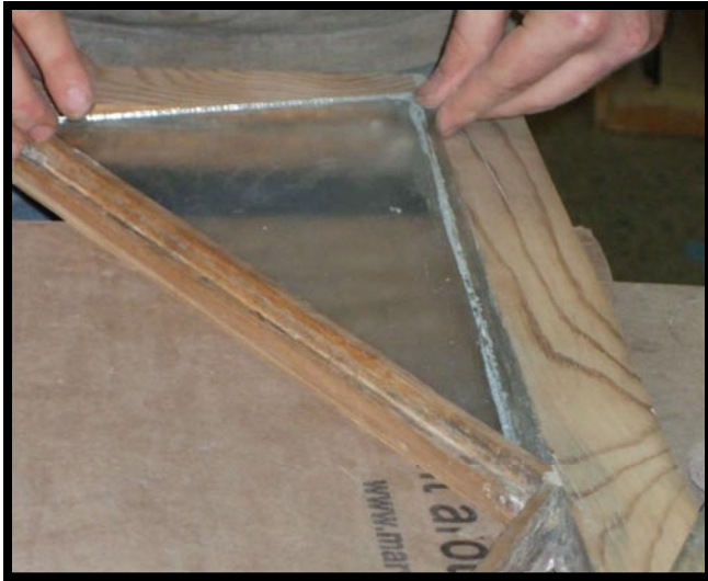
42.) Glass panes test fitted.
