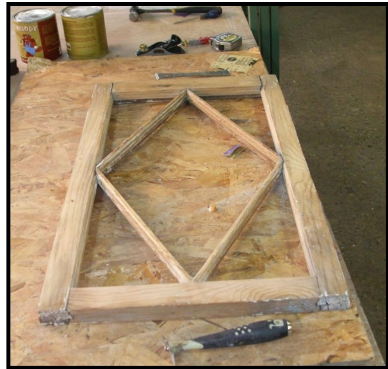
23.) [Day 2] Much of the paint has been removed.
