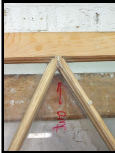
56.) Previous adhesive repair after curing overnight.
