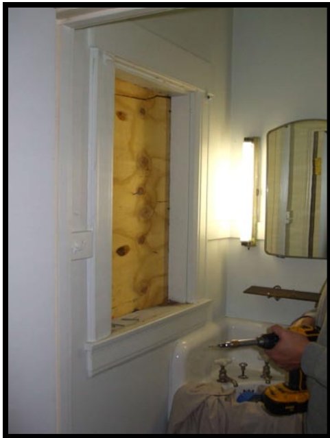
7.) Plywood is installed temporarily with drywall screws driven into the jamb. Painter's tape was applied to prevent air infiltration.
