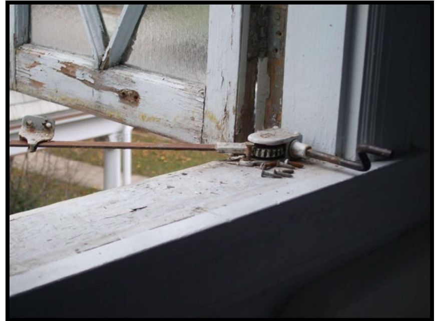
3.) 2 nd floor casement sash operator
