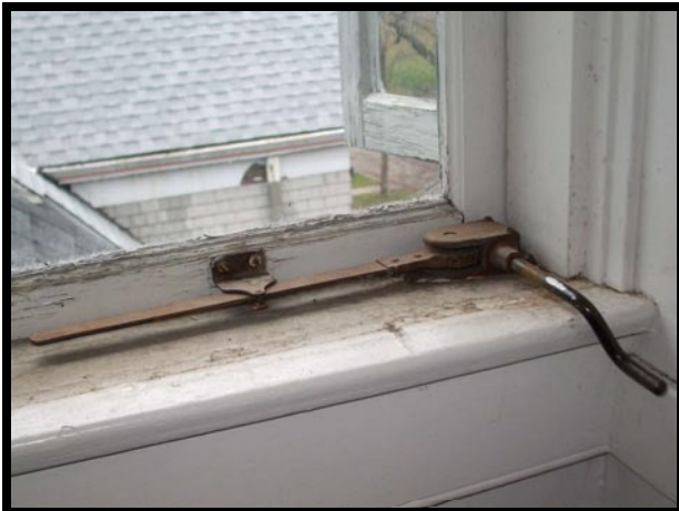
4.) 3 rd floor casement window sash operator
