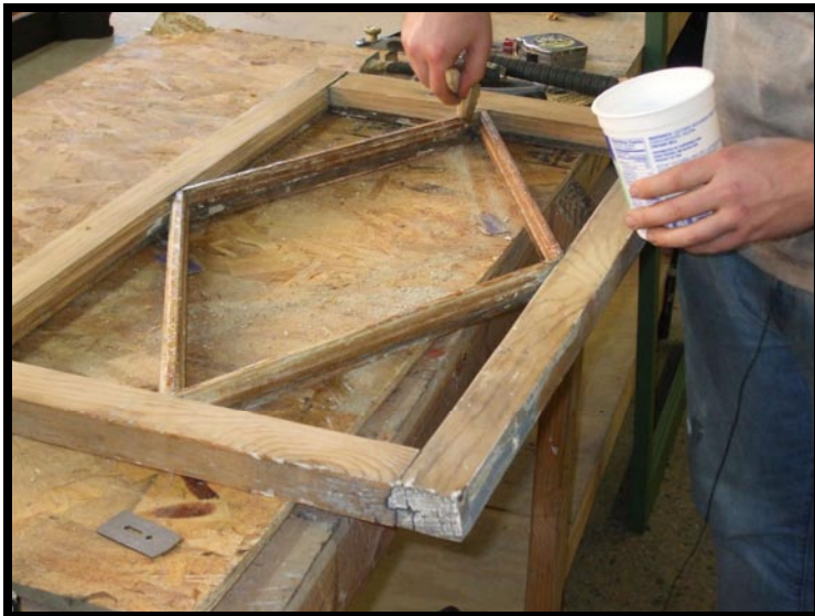
27.) Paint remover applied to aid in scraping paint from the window muntins.
