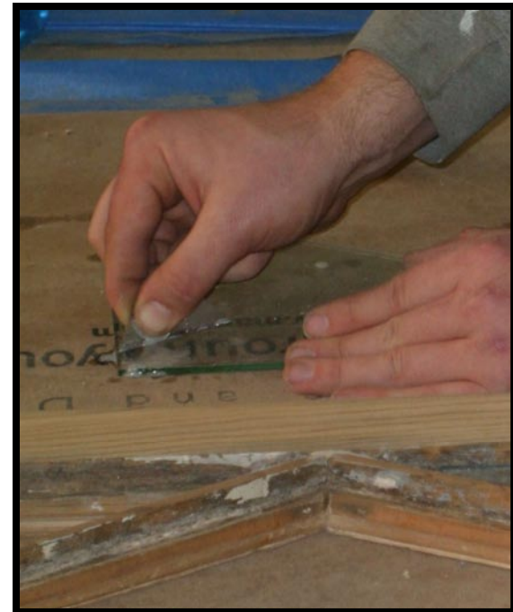
44.) Glass cleaned with window cleaner and a straight razor.
