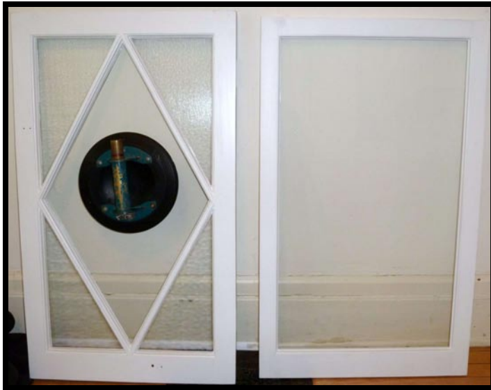
62.) A Wood's Vacuum Cup is being used to install the restored sash. An interior storm window is on the right in this photograph.
