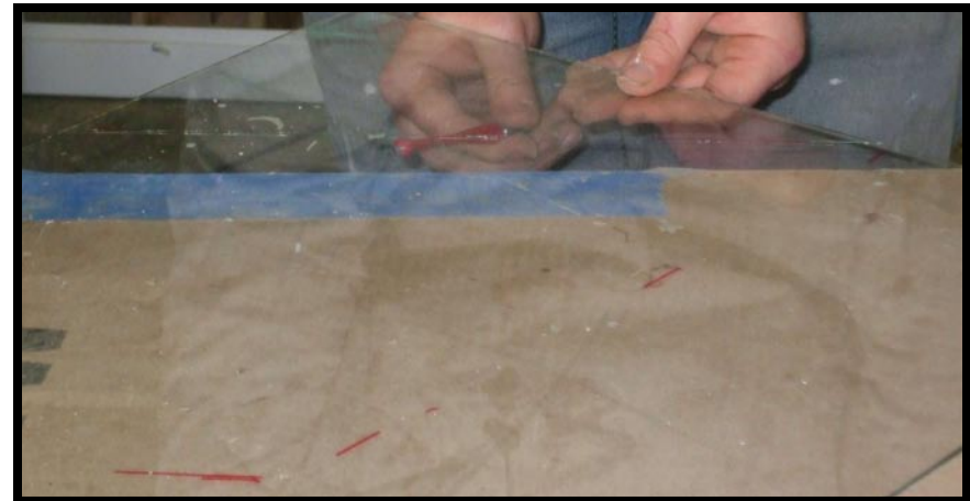
52.) Cutting a new center pane.
