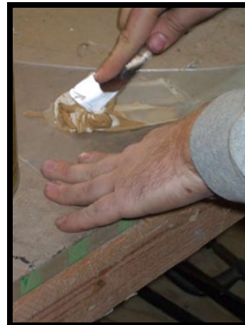
31.) Mixing equal parts of the wood epoxy.
