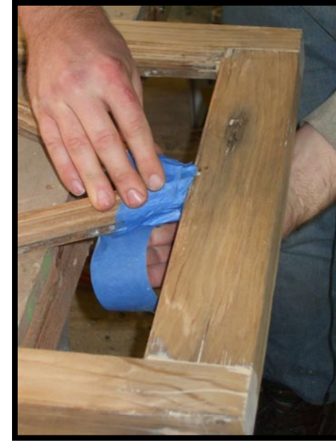
39.) Loose muntin repair: an adhesive is applied, and the joint is clamped with tape.
