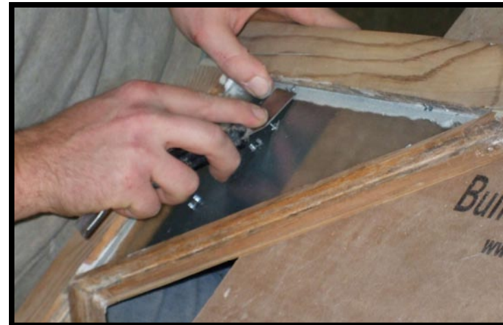
46.) Glass pane installed over glazing compound bead; glazing points installed.
