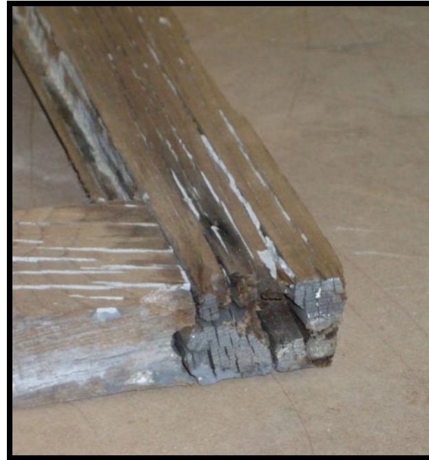
29.) Rot, deterioration on 3 rd floor casement stile.
