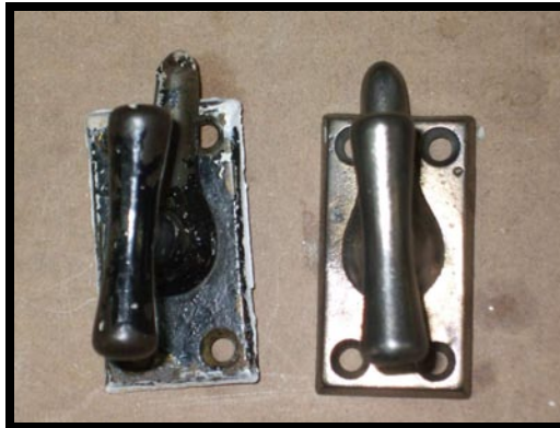
61.) Window latches prior to final paint removal with a wire wheel and after using the wire wheel on the bench grinder.
