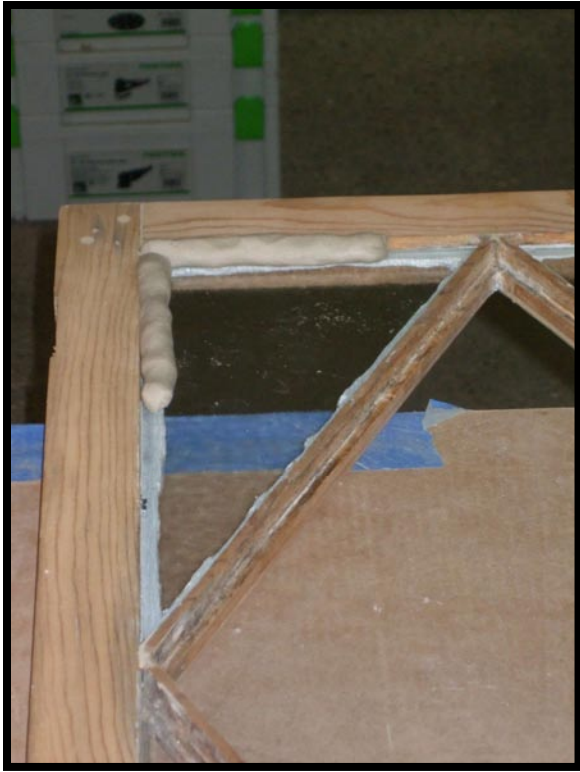
47.) The glazing compound is kneaded, rolled up and placed over the glass and glazing points.
