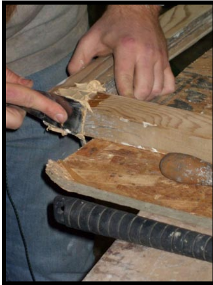
32.) Applying epoxy filler to the 2 nd floor casement sash stile end grain.
