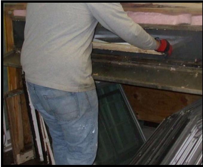
22.) Sash placed back in the steam box.
