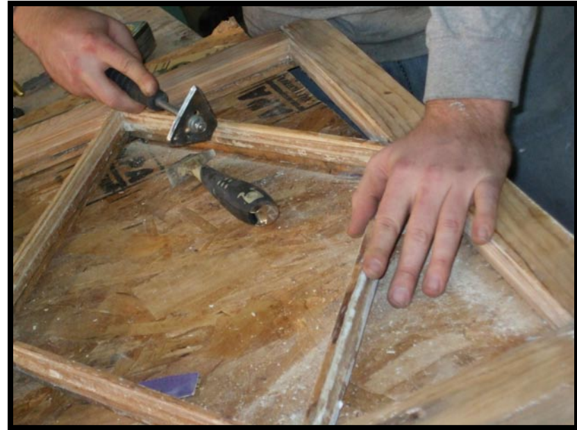
26.) Scraping paint from the window muntins.
