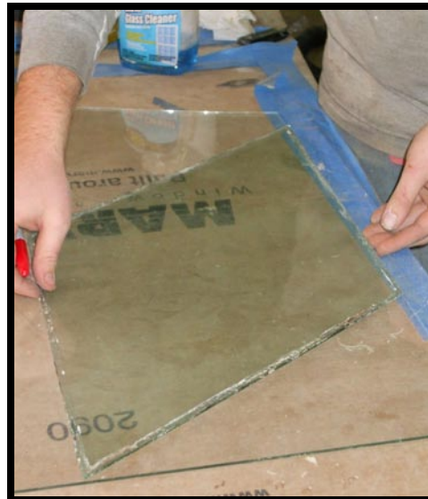
51.) Cracked center pane for the casement dimensioned for replacement.
