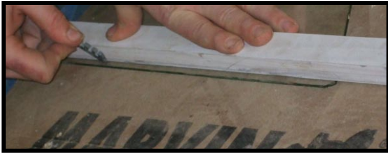
53.) Center pane is trimmed to fit 2 nd floor casement muntins.
