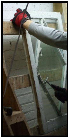
19.) Paint and putty scraping, removal.
