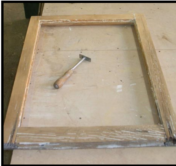
25.) 3 rd floor casement after steaming and scraping.
