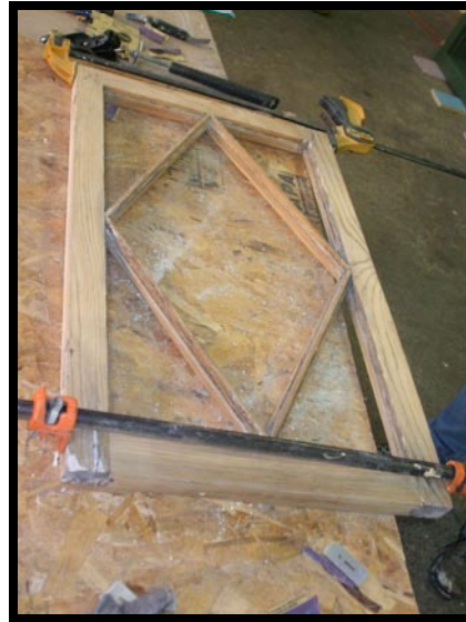
33.) Clamps placed around the frame while epoxy dries.
