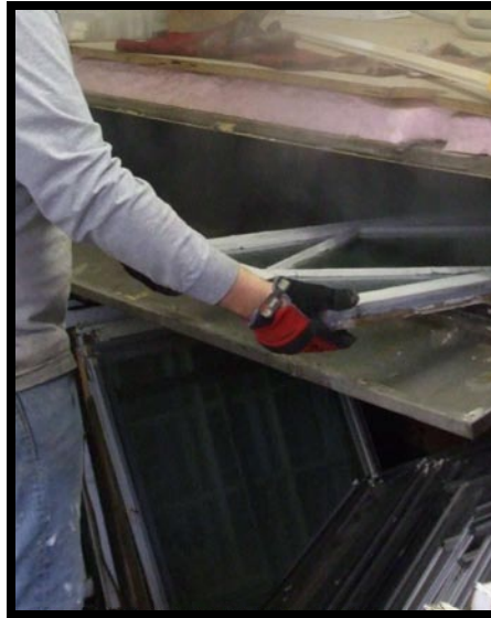
17.) Window removed from the steam box.
