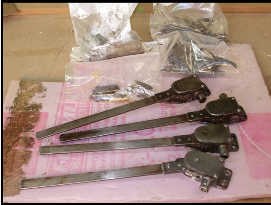
58.) Casement operator hardware and sash hardware undergoing cleaning and lubrication.
