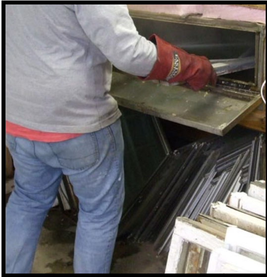
16.) Window placed in a steam box.
