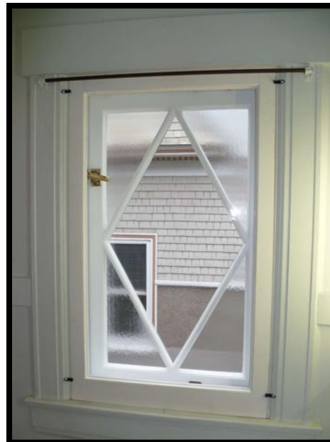
64.) The interior storm window is installed. Tabs at each corner hold the storm window in place. The casement operator crank has been removed and stored for the winter.
