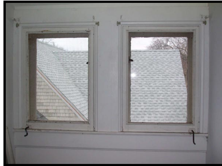
9.) 3 rd floor casement windows.
