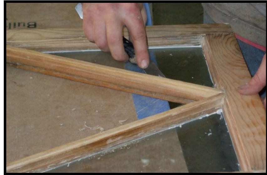
50.) Opposite face of glass cleaned of excess latex glazing compound.
