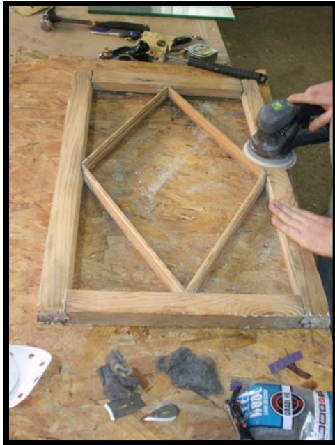
28.) Orbital sanding with HEPA vacuum attached.
