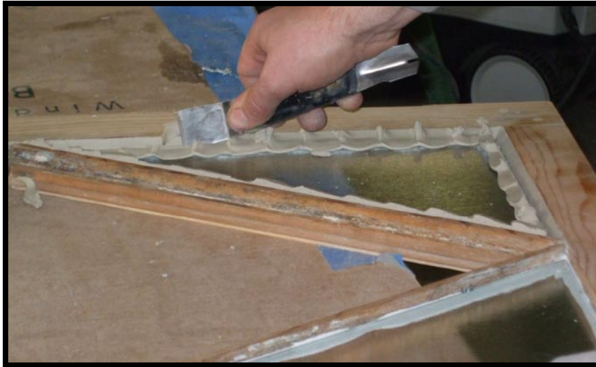
49.) Glazing putty cut to profile with a putty knife.
