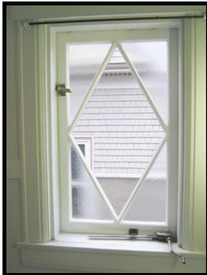
63.) The restored casement window is installed.
