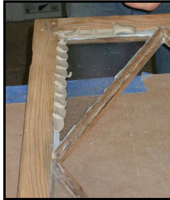
48.) Glazing compound pressed into muntins, rail, stiles with a putty knife.
