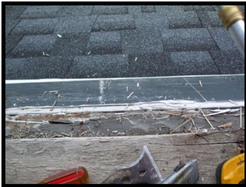
13.) Rot at 3 rd floor sill. A partial earlier repair by another contractor was discovered.
