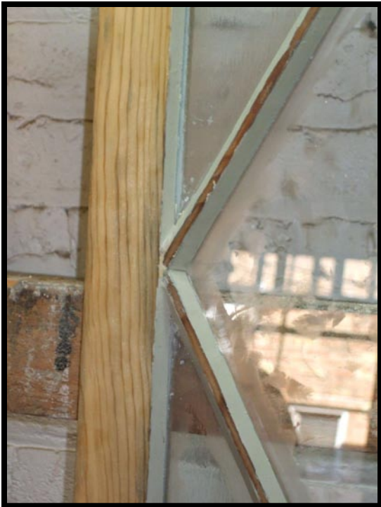
55.) [Day 4] Glazing completed. Profile of glazing putty.
