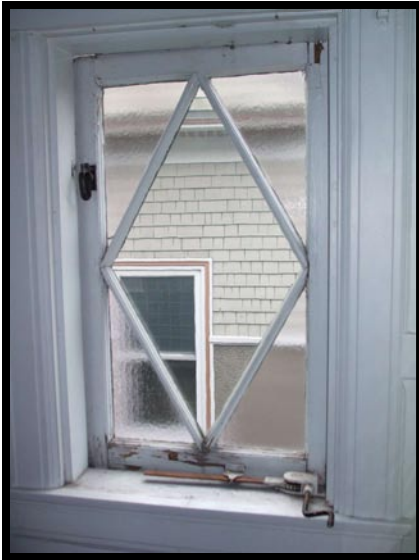
1.) 2 nd floor casement window prior to removal.
