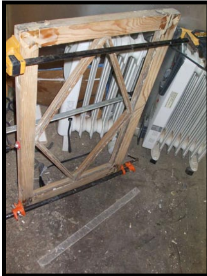
35.) 2 nd floor casement sash left to dry in the “heat room”.
