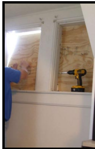
14.) Plywood panels installed following removal.
